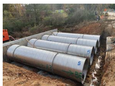
Culvert Construction- First Stage
